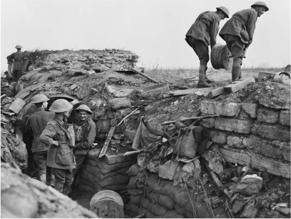
AWM E00798. Signal Engineers, with a reel of cable to lay a surface telephone line to a forward unit. Buried cable routes were mainly relied on, but when these failed through shellfire, surface lines were run out as a temporary measure until communication by the buried lines was restored.
