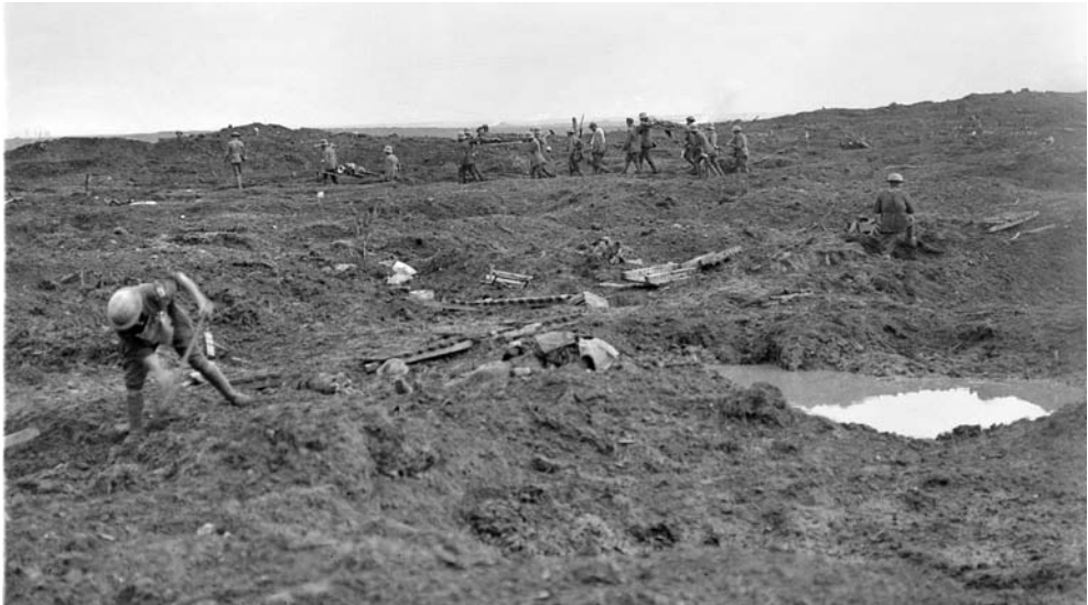
AWM E00747. Signallers laying a line of telephone cable.
